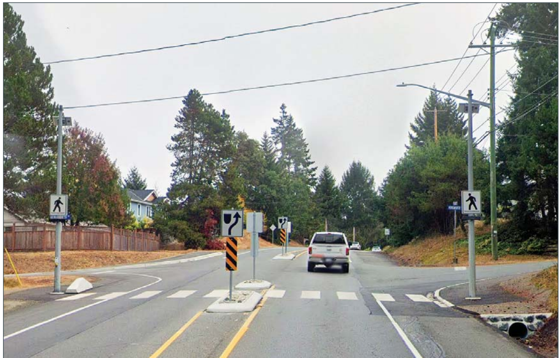
Figure 2.3 – Median islands at Hemsworth Road
